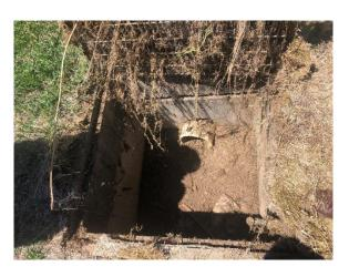
Plate 6.10 A drainage systems within the base of the velodrome
