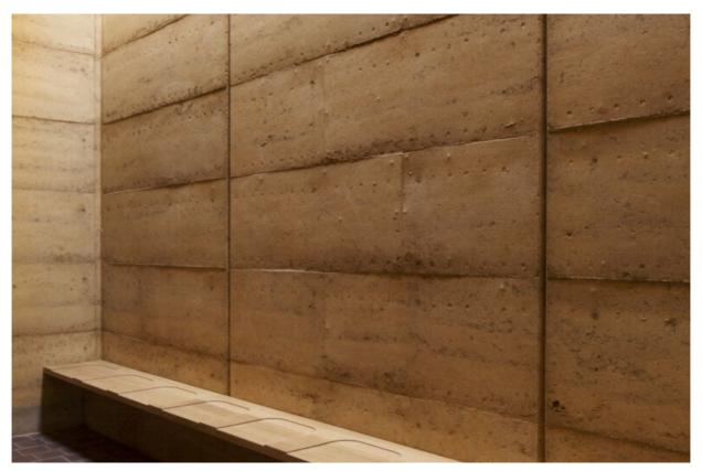
Figure 25. Detail of the rammed earth at the Bushey Cemetery | Elliot Wood
